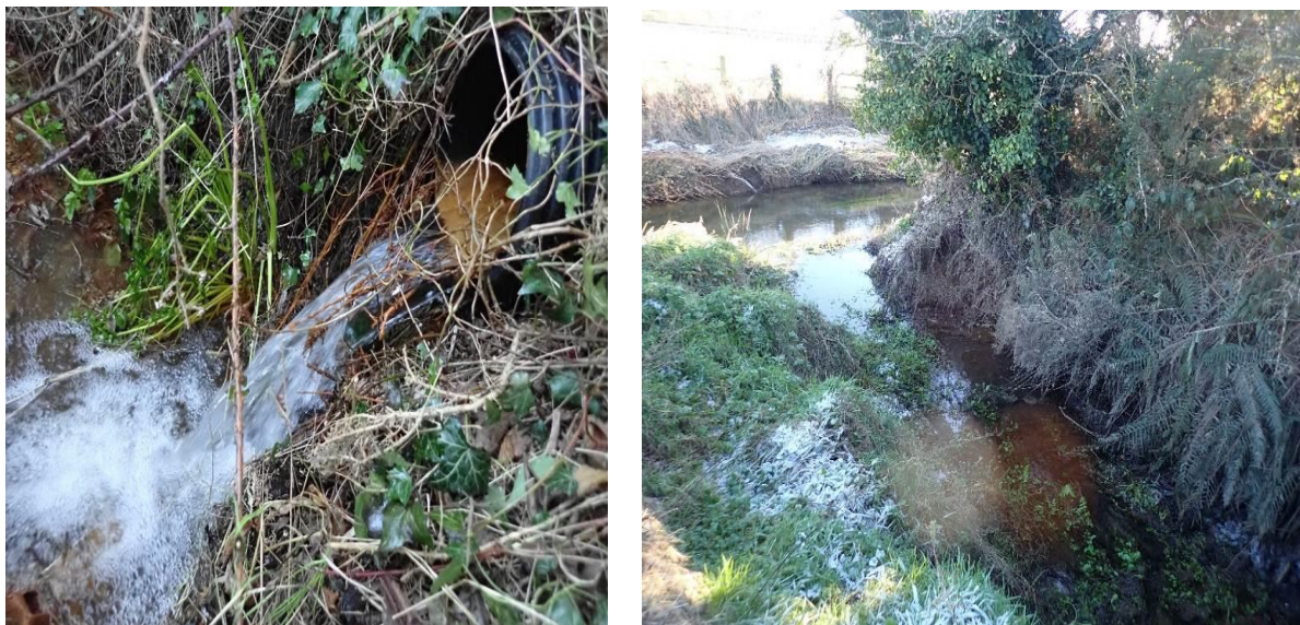
Figure 3 Corrugated plastic pipe discharging water to drainage ditch (left) and drainage ditch at the Tinnacross stream confluence (right)
